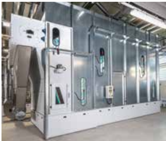
Blending chamber with component-independent blending system
